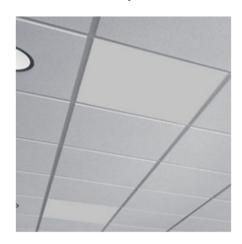
The ceiling panels have a zero fire rating. Their lightweight characteristics make them an excellent option for grid systems without introducing excessive loading.
